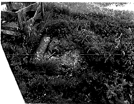
Excrement at septic tank rodding eye
