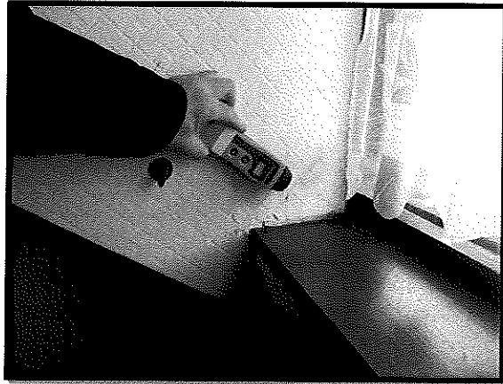
Figure 10 Bedroom 2 damp stain
