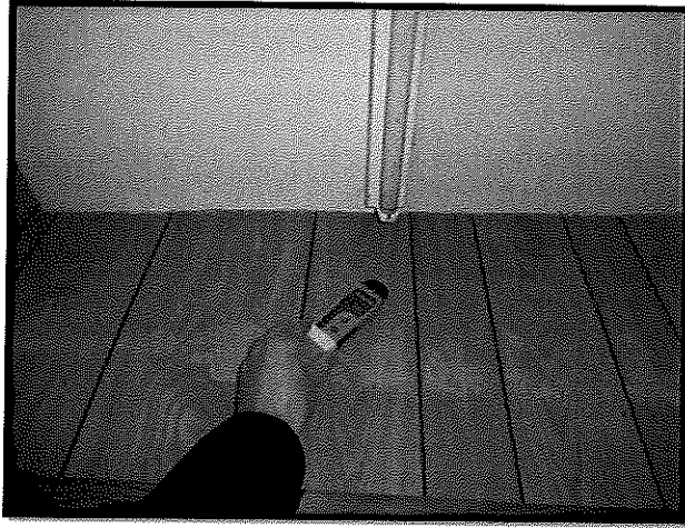
Figure 6 Rear Extension residual damp
