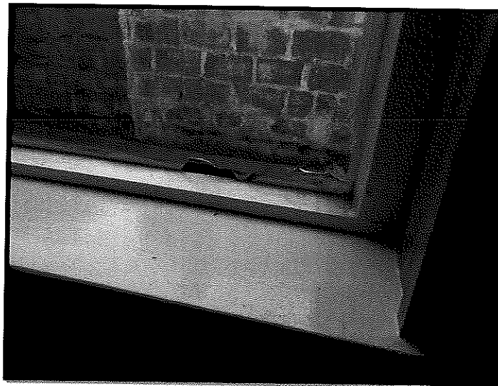
Figure 5 Rear Extension holes in glazing
