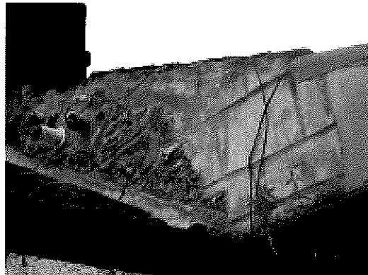
Rear roof skew
