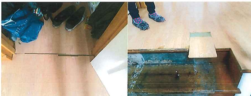
Laminate floor to landing
