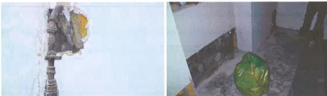
(Ph3) FE – Base. Bed. exposed p/work (Ph4) FE – Base. Bed. exposed tanking
