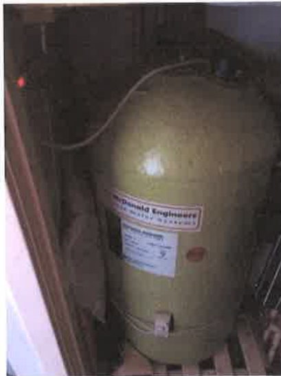
Immersion heater and hot water cylinder tank
