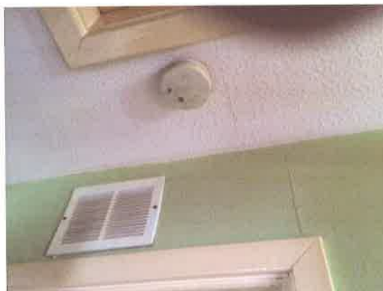
Inner hallway - battery operated smoke detector
