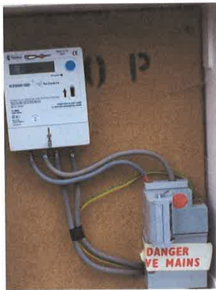
Meter cupboard – electric pre-payment meter
