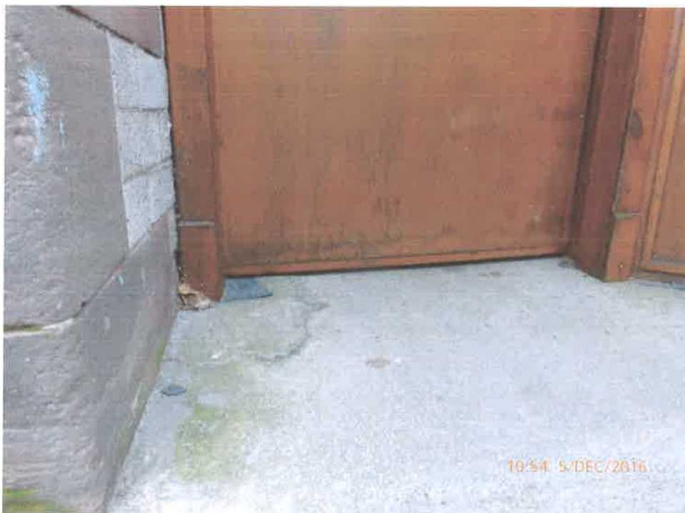
Gap below front door and door not closing
