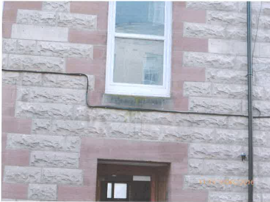
Evidence of past rainwater spillage
