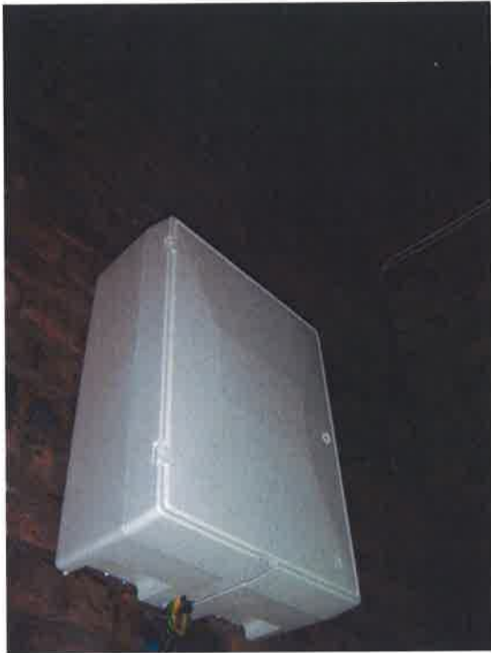
New Upvc Electrical box fitted
