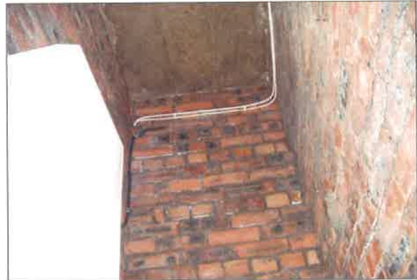
Coal Cellar under external stair
