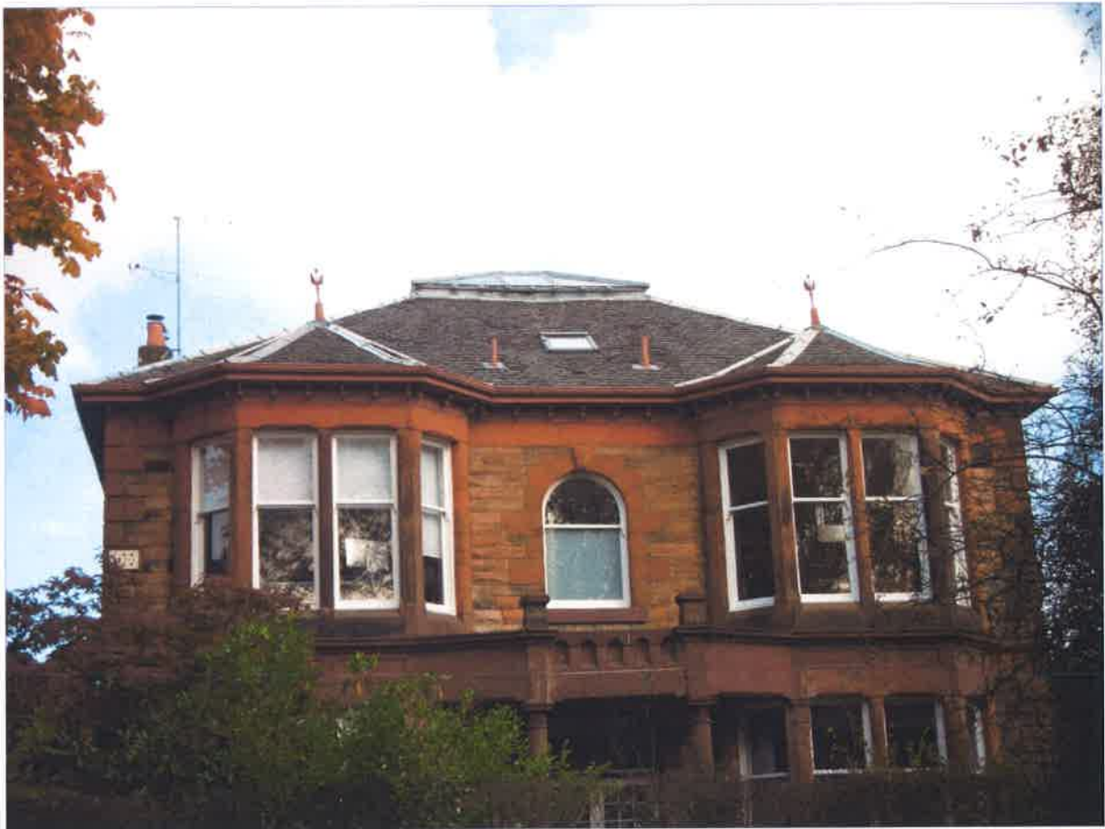
Front elevation - visible from ground level roof undulation/sag, missing, slipped and broken slates.
