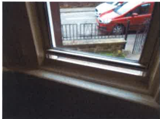
Living Room - bay window - Internal - right side
