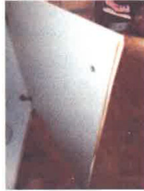
Kitchen - base unit door to right side of oven - outer coating peeling
