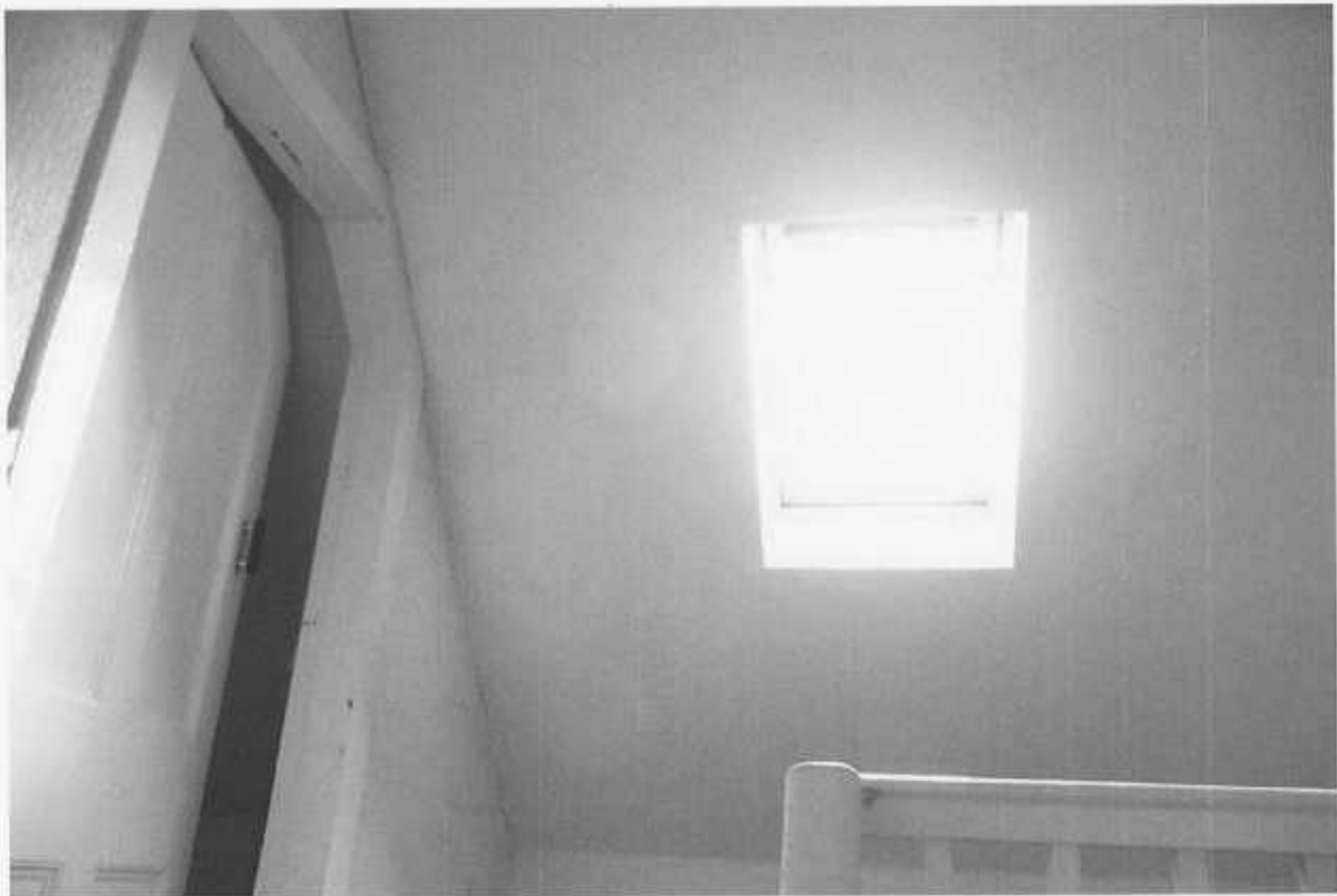
Top floor landing ceiling (former hole)
