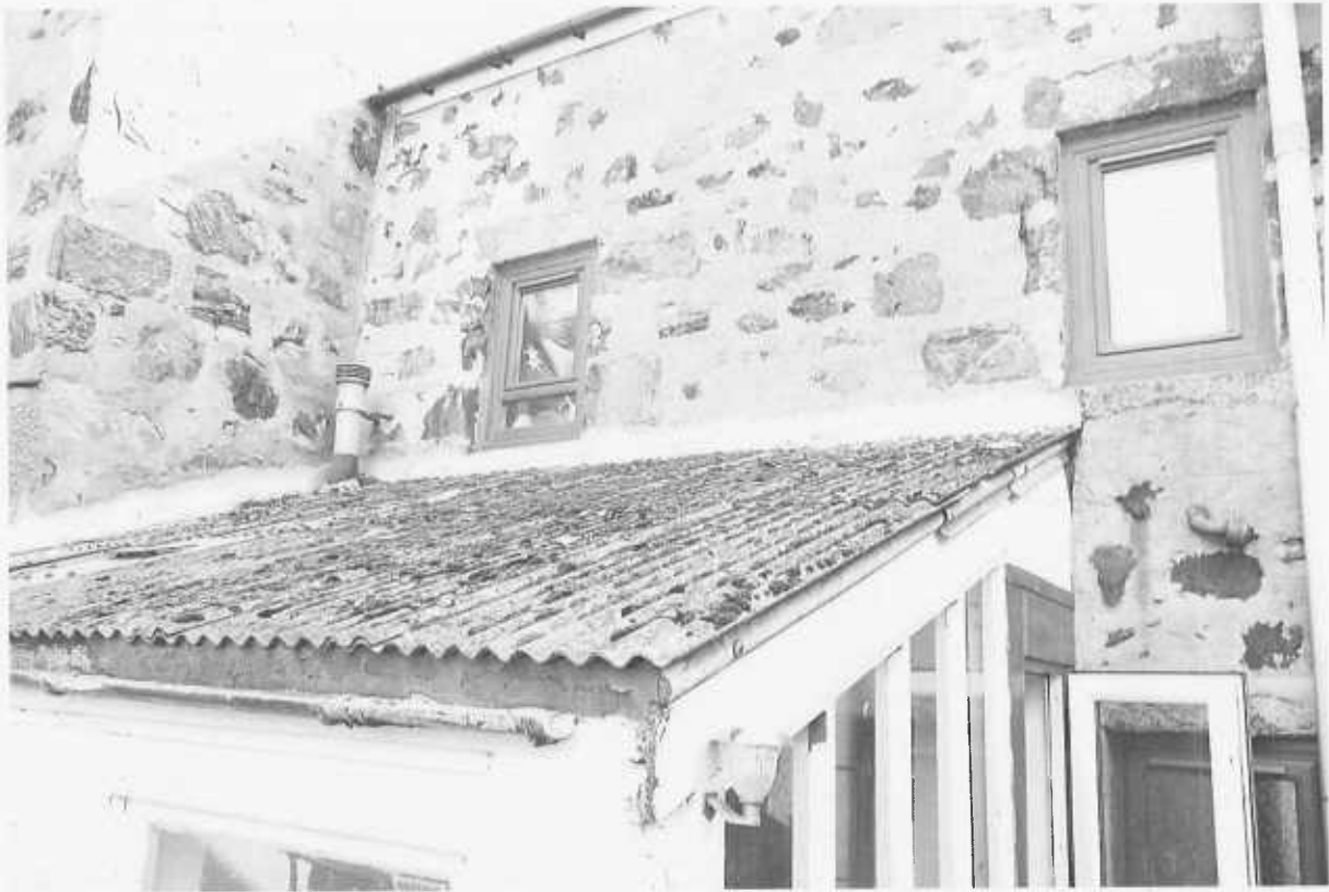
Rear porch roof post repair
