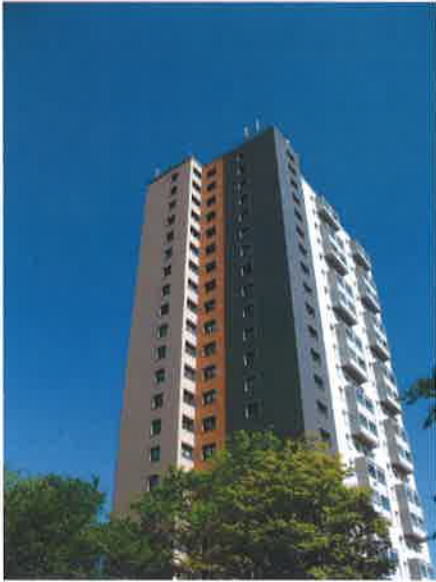
01 - Front elevation (Flat 85 is 18th floor, front corner)
