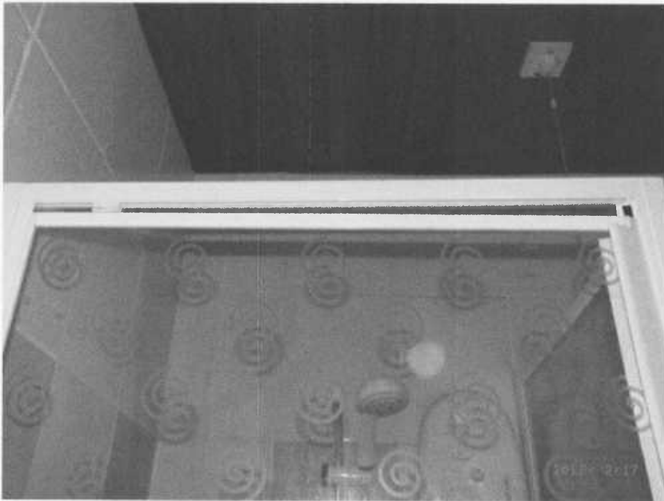
Shower enclosure alignment
