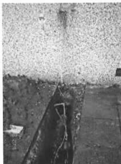
New/old feed supply For central heating
