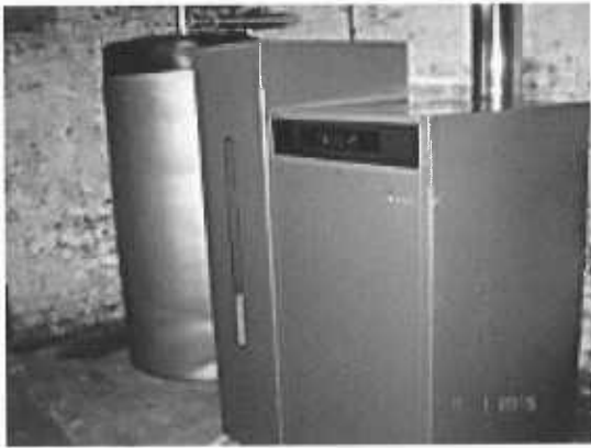
New central heating plant
