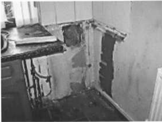
Location of former oil central heating boiler.
