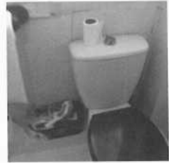
16. Bathroom WC Unit
