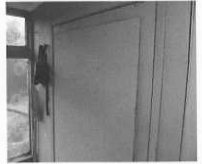
7. Kitchen Porch Back Door
