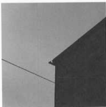
19. Cast Iron Gutters
