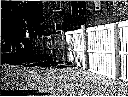
New fence/gravel area
