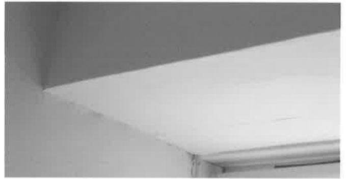
3b) As at 1/09/16: kitchen ceiling repaired
