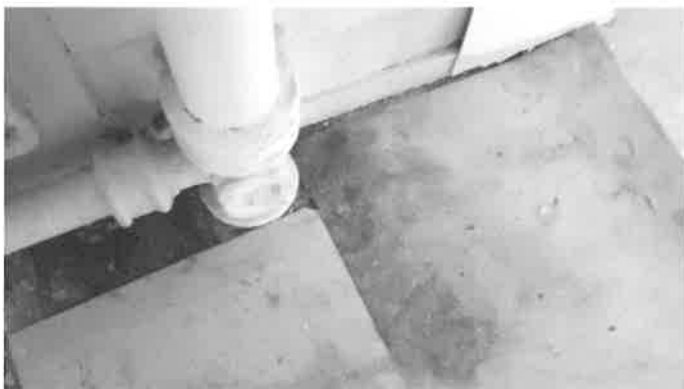
4a) Kitchen floor at 5/08/15
