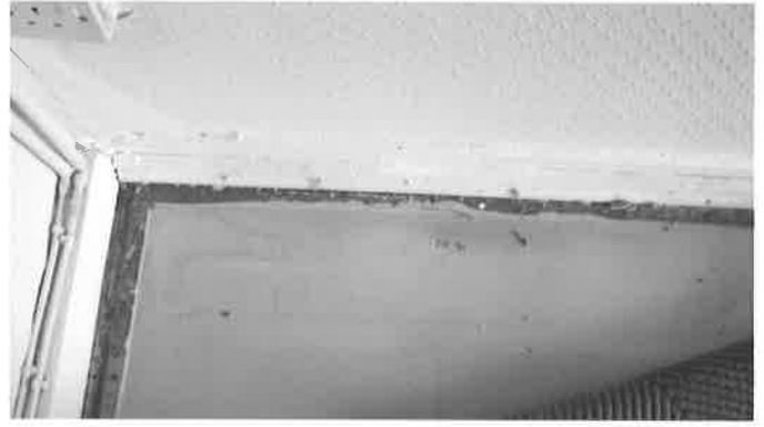
2d) & 2e) As at 1/09/16: evidence of new screed and carpet underlay
