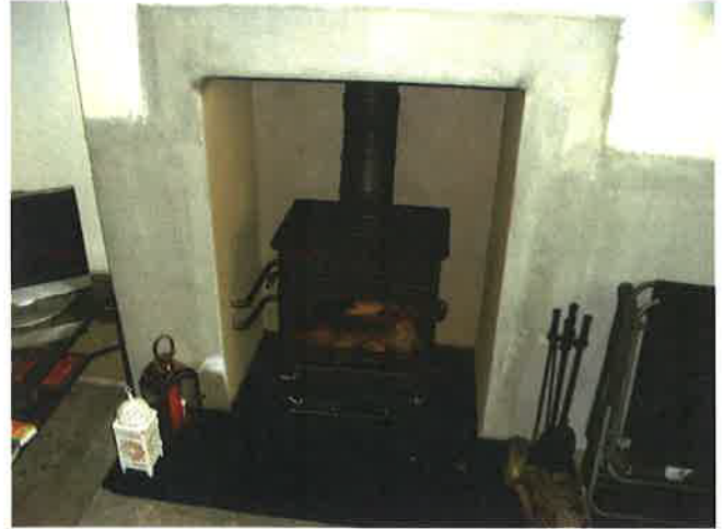
02 – New multi-fuel stove (with new back boiler)
