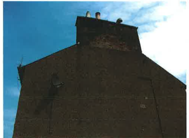
04 – Gable wall (roughcast except for chimney head)
