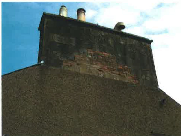
05 – Chimney head (part brick & part stone block)
