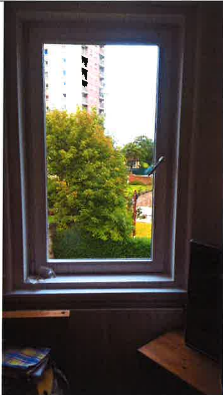
Rear bedroom window replaced and made good.
