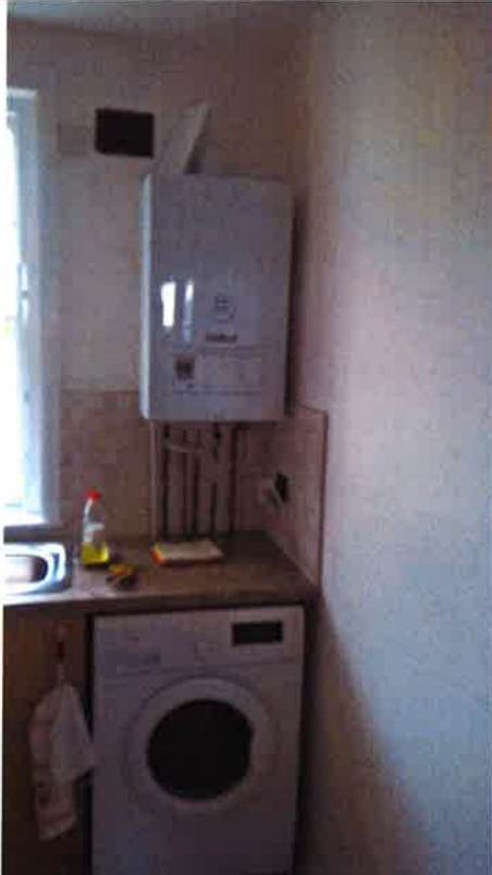
Kitchen. Walls re plastered and decorated.
