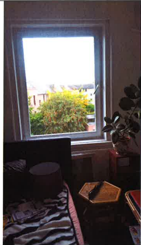
Front bedroom window repaired and made good.
