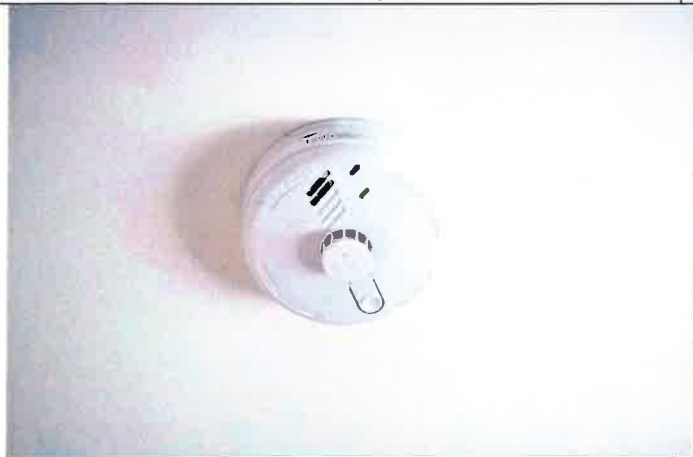
Hardwired heat and CO Sensor installed in kitchen
