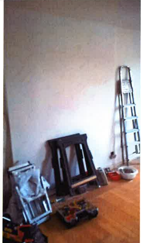
Living Room. Redundant fireplace removed and opening made good.
