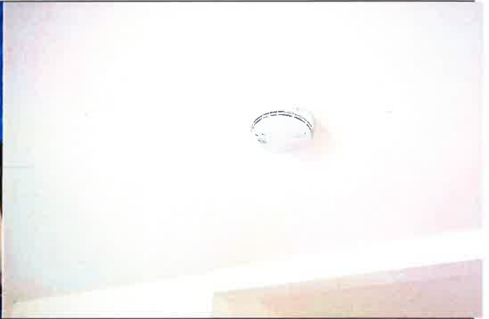
Hard Wired Smoke Sensor installed in living room
