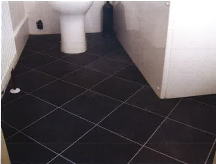
2: Replacement bathroom floor covering
