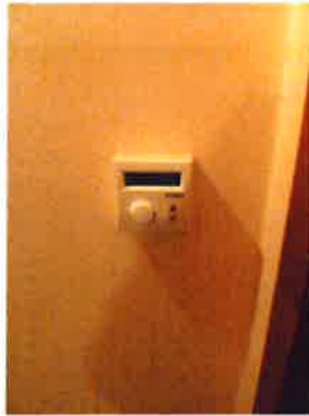
6. Central Heating Thermostat /Programmer
