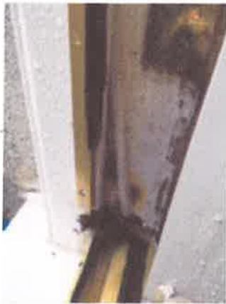
Front Porch Door - internal view showing gap in draught excluder
