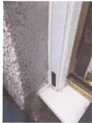
Front Porch Door - external view of lower section - gap in draught excluder
