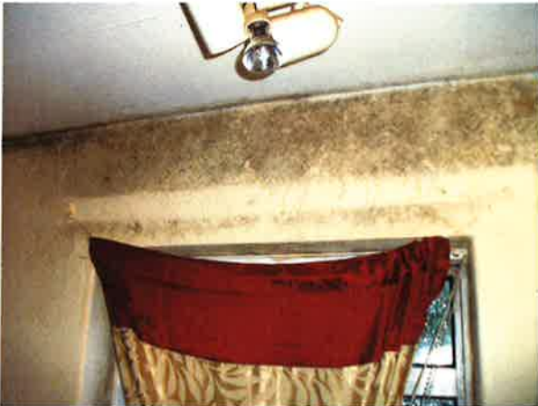
09 – Wall above stair window
