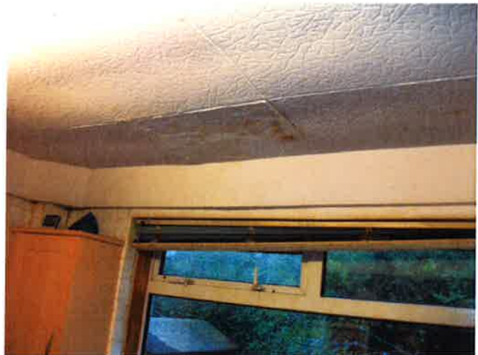
04 – Kitchen ceiling at window
