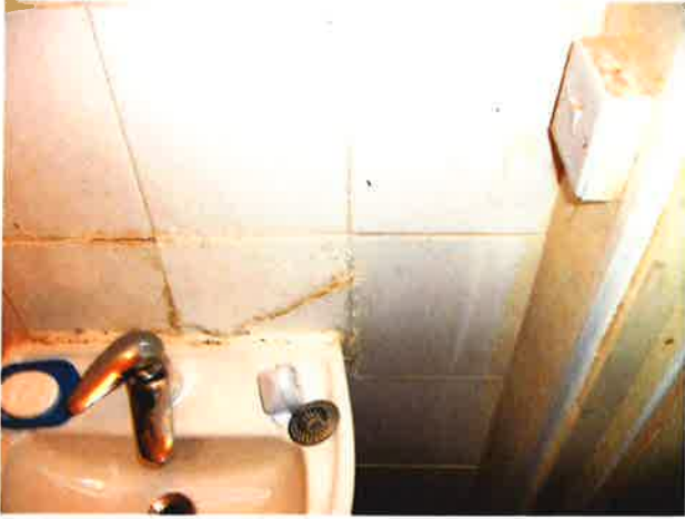
27 – WC & WHB (under the stairs) – light switch
