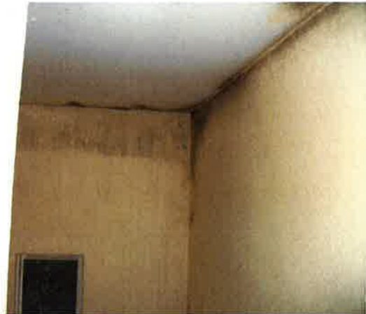
10 – Stair well (left of stair window)
