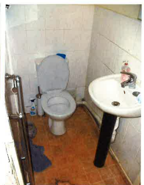
07 – Toilet (under stairs)
