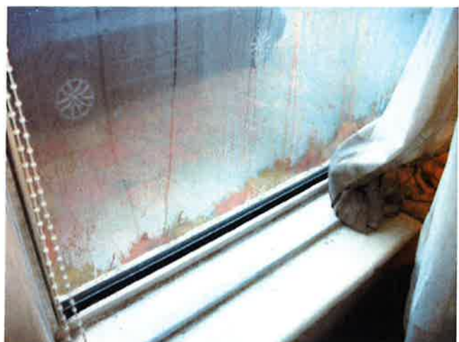
06 – Ground floor Bedroom window (gable)
