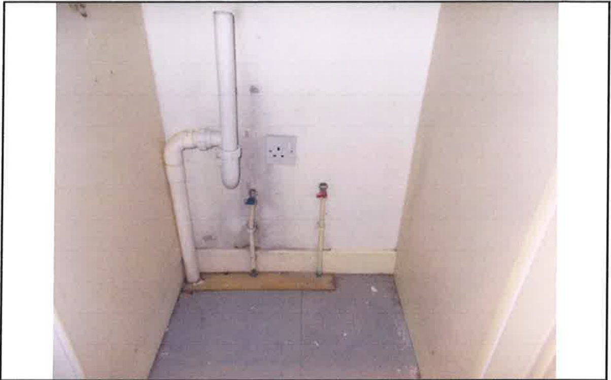
1. Pipework for washing machine 24 May 2017
