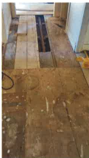
18) Laminate flooring: removed in hall. Damaged sub-floor makes floor unstable
