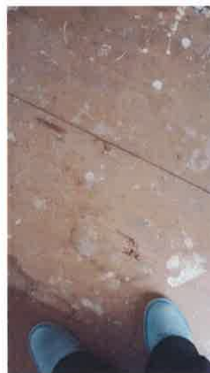
18) Laminate flooring: removed in hall. Damaged sub-floor makes floor unstable
