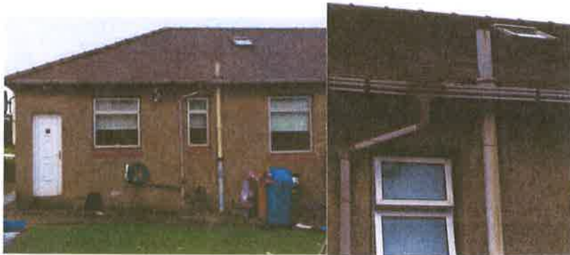
Rear elevation 19 January 2016
