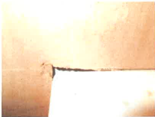
Bathroom - end of bath at external wall
