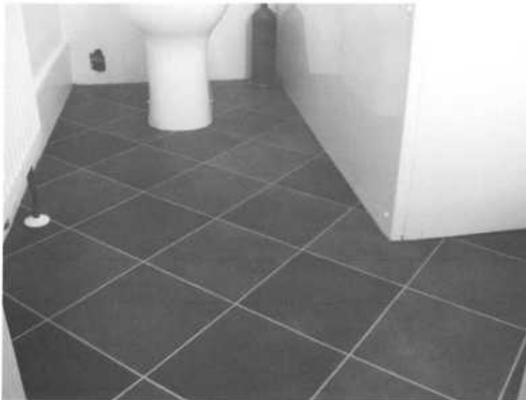
2: Replacement bathroom floor covering
