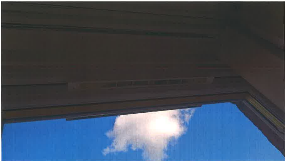
9. Closed trickle vent to Bedroom with mould growth.
