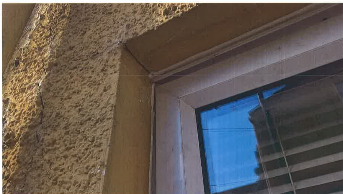
2. Kitchen window sealants and crack to render.
