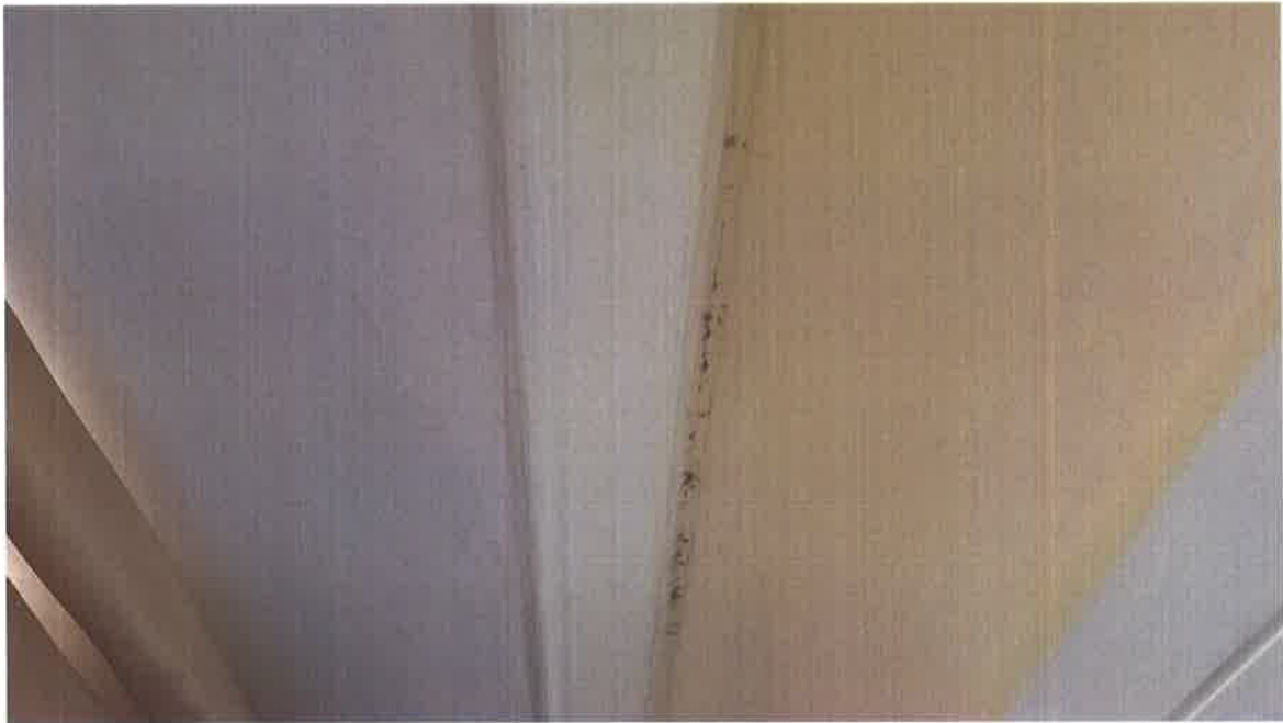
11. Area of mould contamination within Bedroom adjacent to window.
