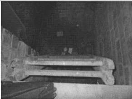
Basement access ladder
