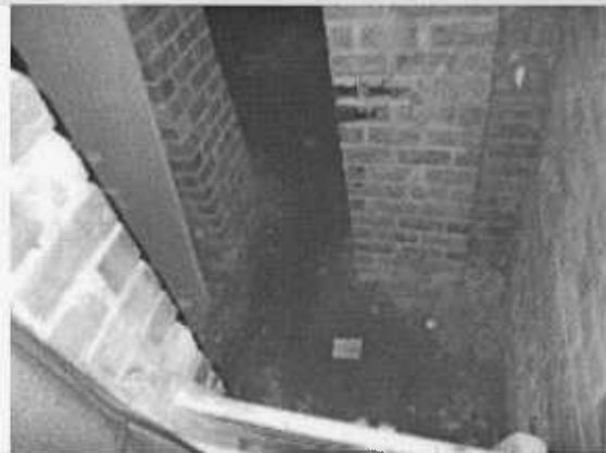
Basement - view from back of cupboard
