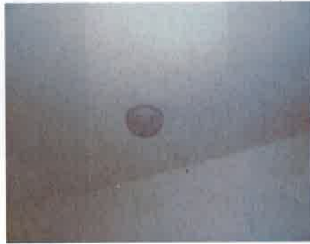
9. Hard wired heat detector
