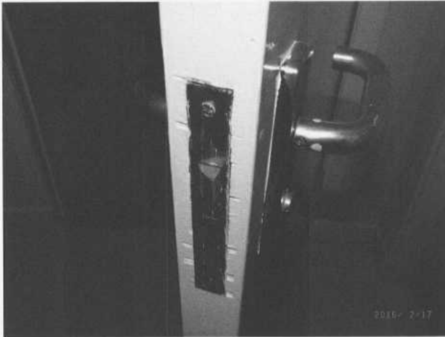
Bathroom door lock
