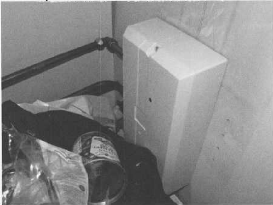
Replacement water heater below Kitchen sink
