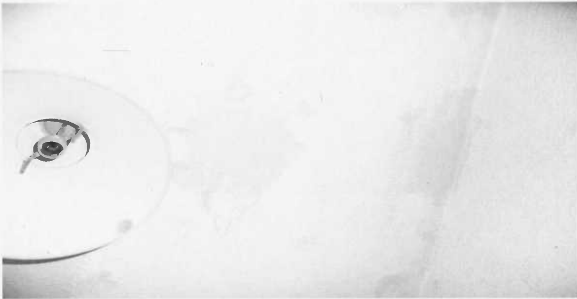
Alleged damp ceiling – due to poor decoration
