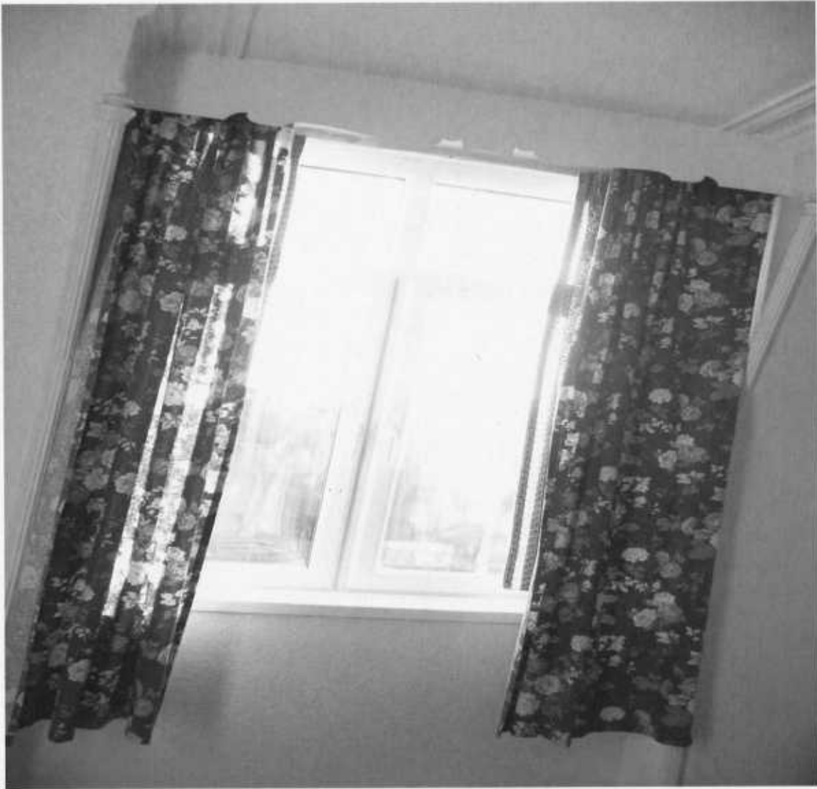
Replacement window in Living room
