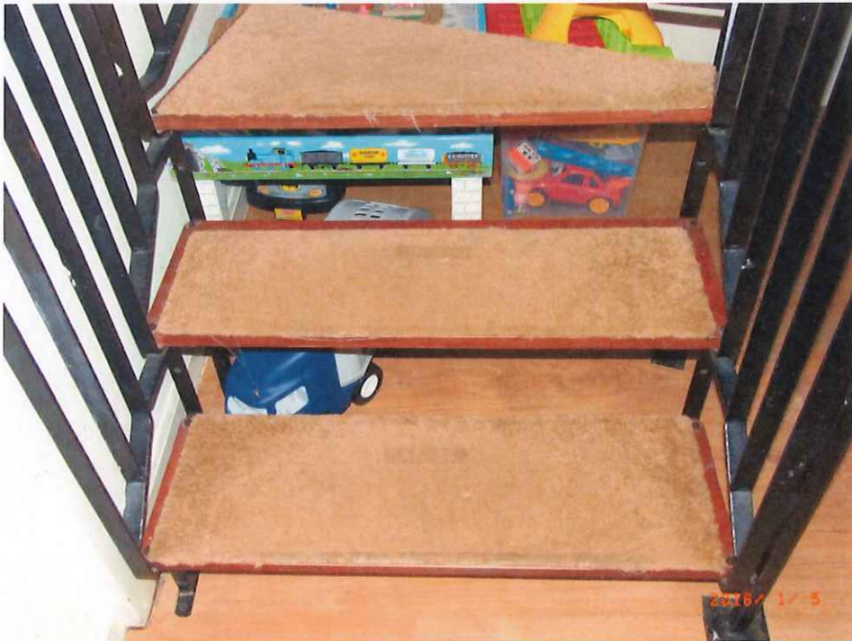
Staircase – typical stair treads
