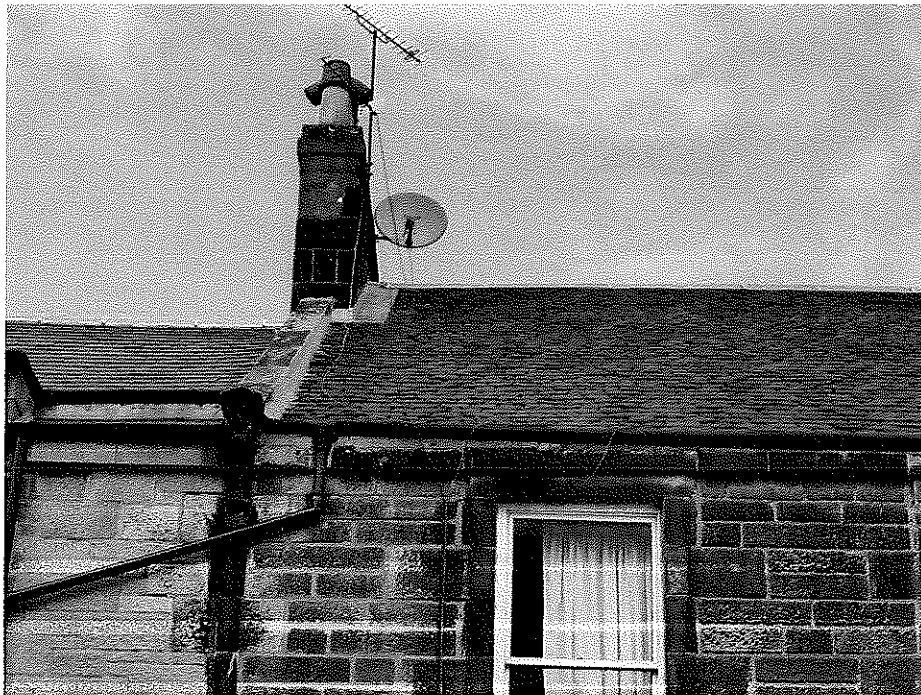
Detail showing repair undertaken
