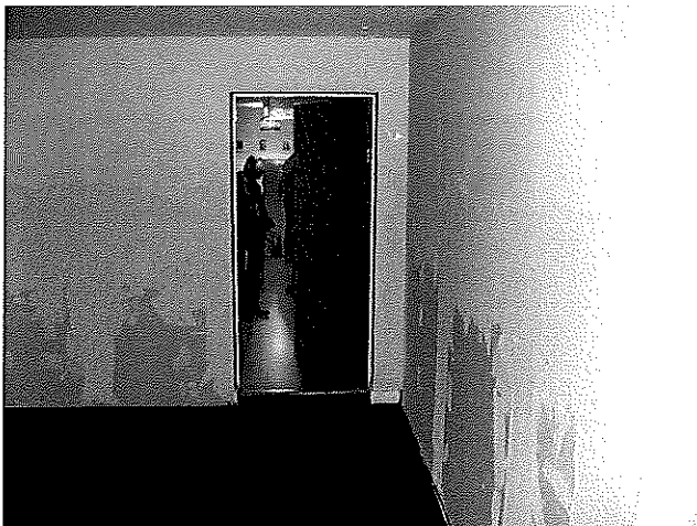
05 - 5 th floor landing (flat 5/1 entrance)
