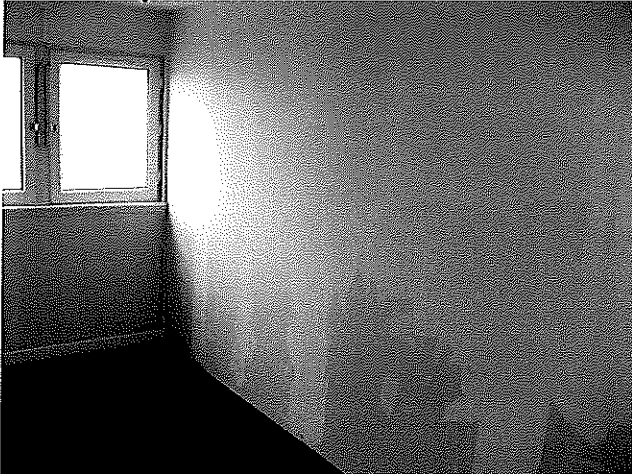
01 - 5 th floor landing (wall of flat 5/1)
