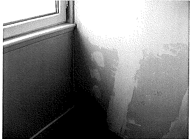
02 - 5 th floor landing (at window)
