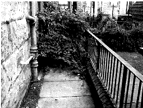
Figure 4 Railings at Rear of Building
