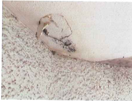
Rear Porch - ceiling
