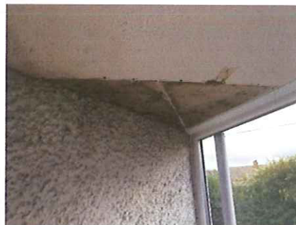
Rear Porch - ceiling
