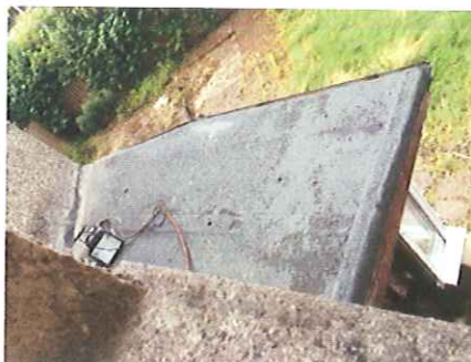
Rear porch - roof
