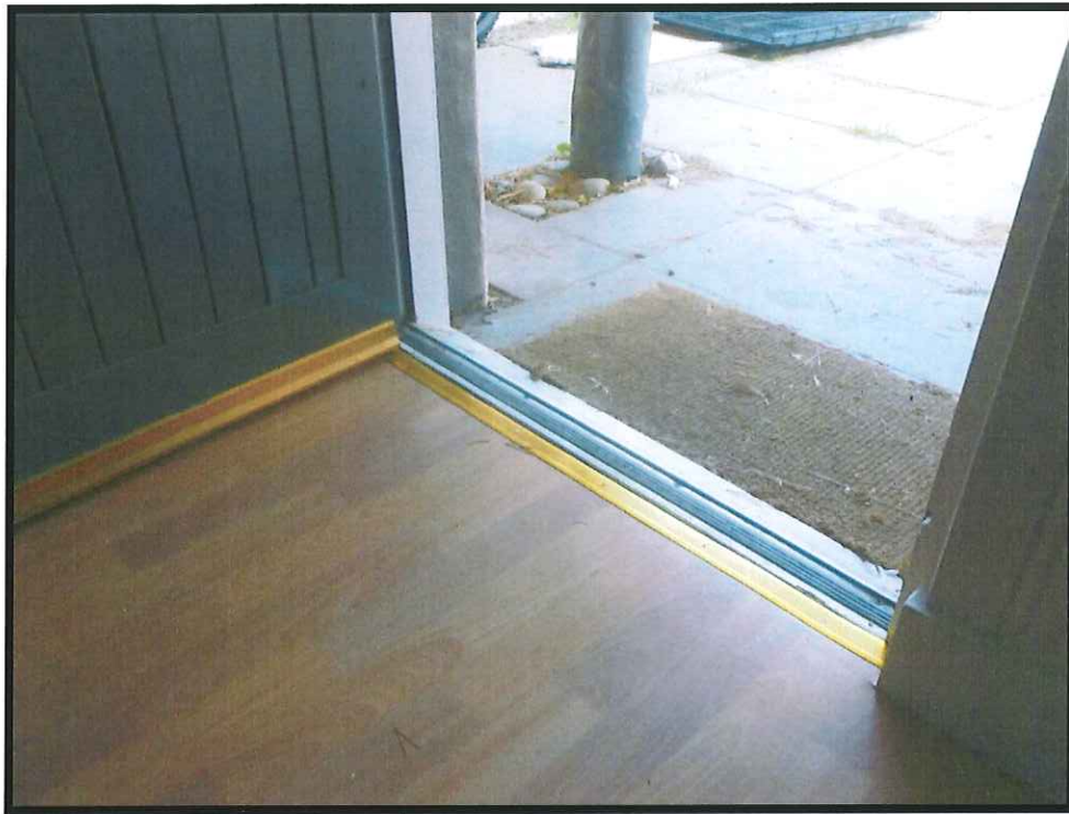
Figure 4 Rear (main entrance) door threshold
