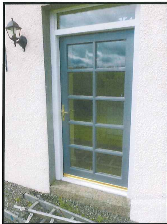
Figure 5 Front door exterior
