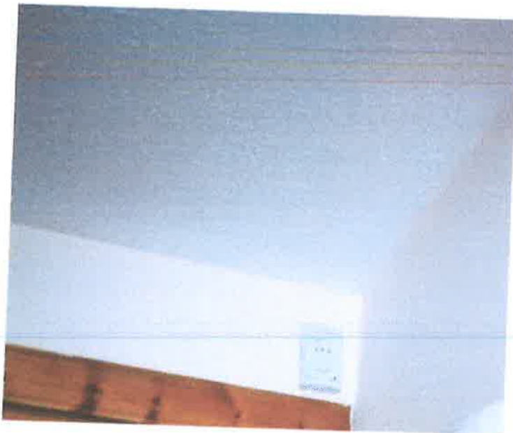
1) CO alarm installed outside boiler cupboard in front lobby
