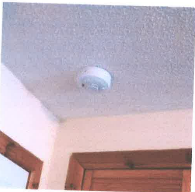
2) Fire detection system upgraded – heat alarm in kitchen
