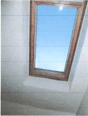
Replacement glazing unit February 2017
