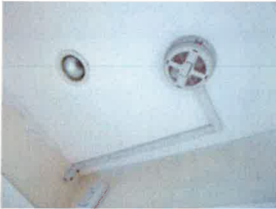
New ceiling mounted smoke alarm in ground floor hall
