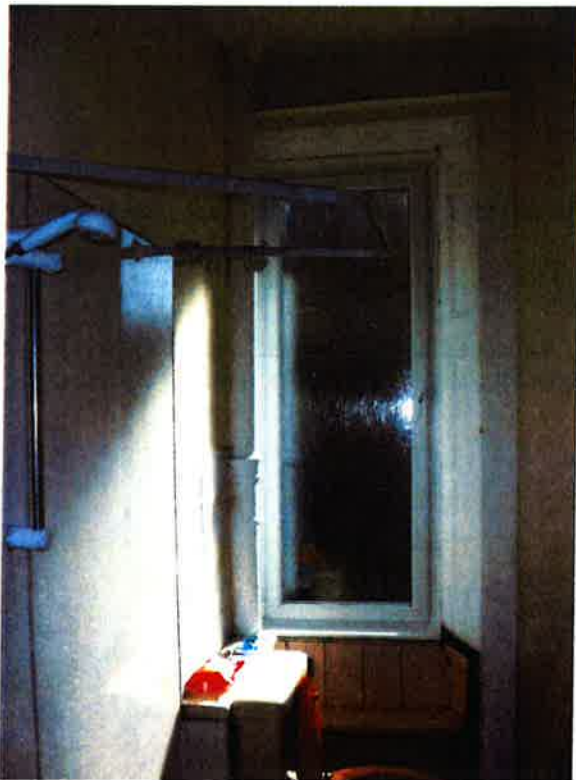
03 – Bathroom window (above front door)
