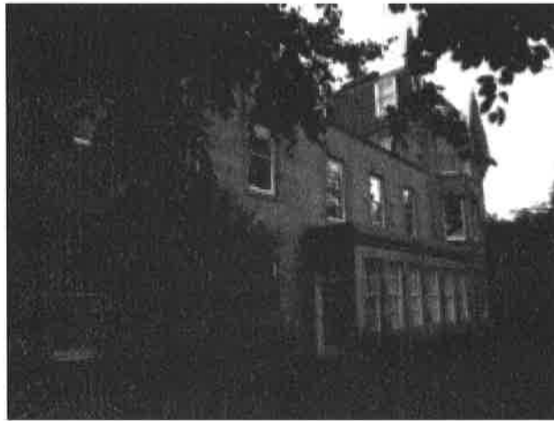
External view - Front elevation of property.
