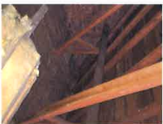
Loft showing where container removed
