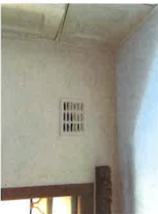
Redecorated ceiling and operational vent
