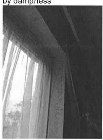
showed previous repairs to render above the bedroom window has been sealed. above window. A projecting 'tray' had been installed above the window - this detail did not occur on any other windows in the development.
