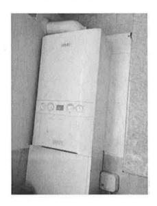
New boiler fitted, Thermostatic Radiator valves & CO Detector
