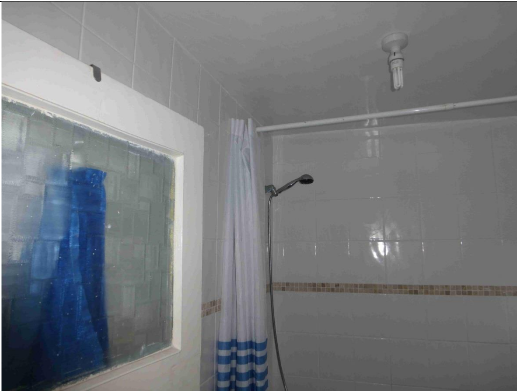
Repaired ceiling in the bathroom
