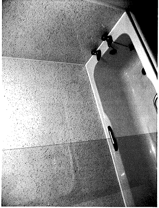
04 - Bathroom -end opposite shower
