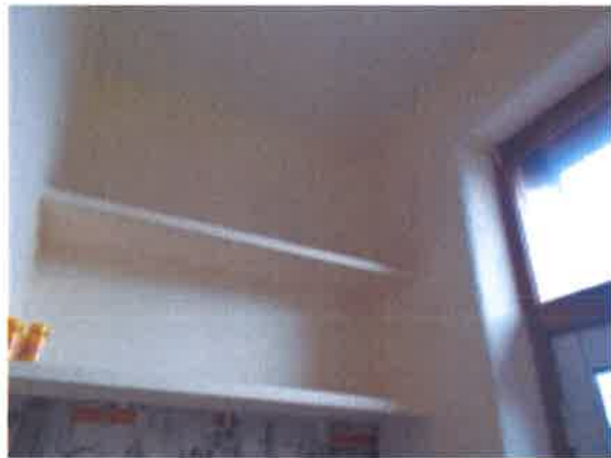
Kitchen - walls re-painted
