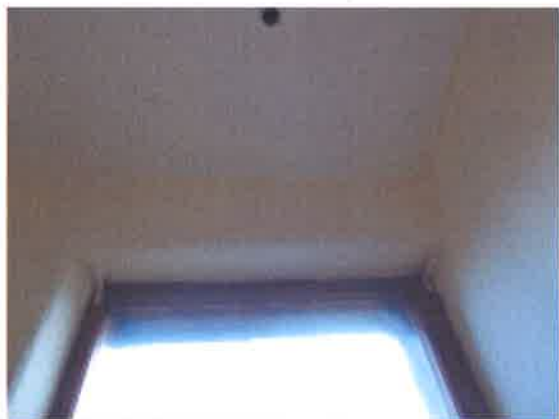
Kitchen - walls re-painted
