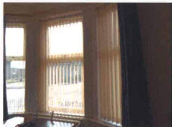
New Living Room Windows - Internal
