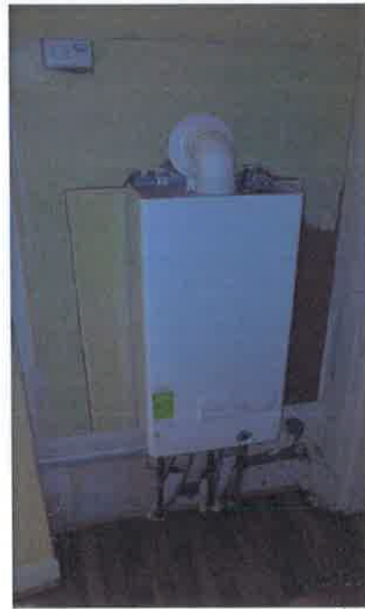
Photo 12 – Gas boiler A Cowan
