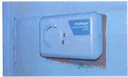
Photo 10 – Carbon monoxide unit
