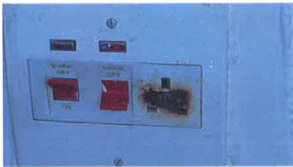
Photo 9 – Damaged socket
