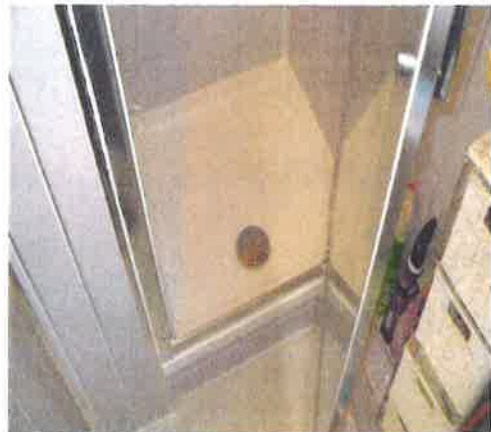
Photo 5 – New shower enclosure
